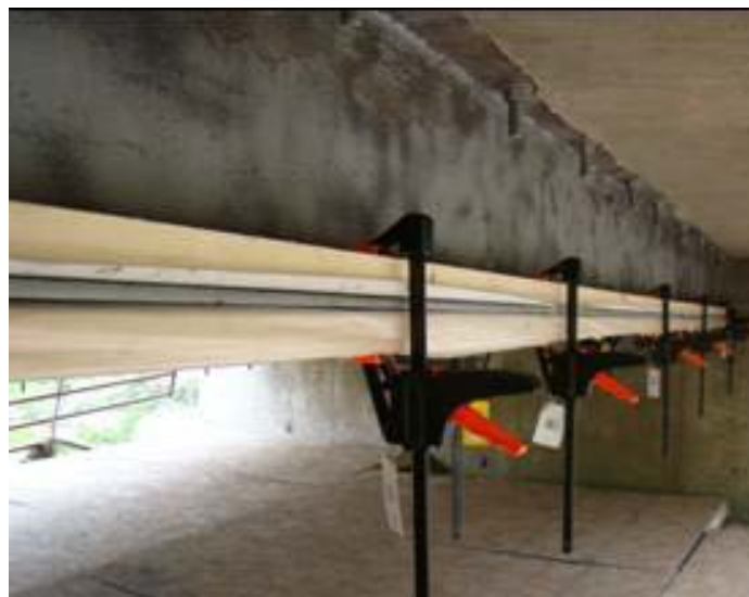
Fig. 5.21: Clamping both top and bottom laminates
