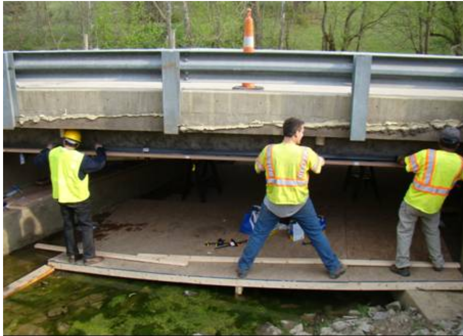
Fig. 5.20: Placing laminate on the top flange
