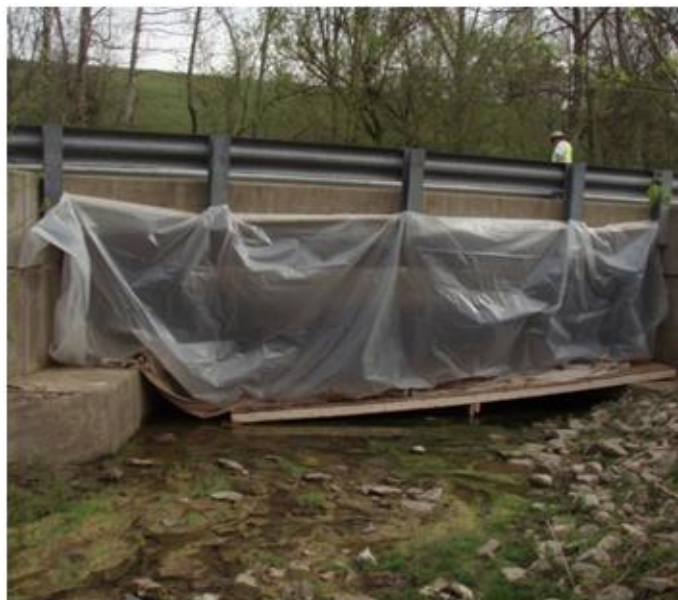
Fig. 5.13: Temporary platform and enclosing for grit blasting
