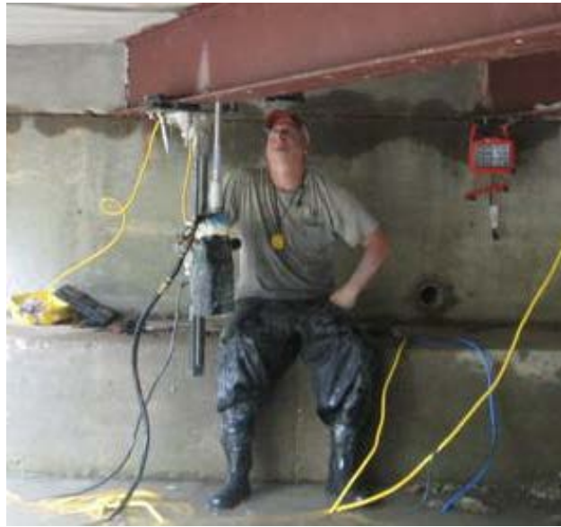
Fig. 5.7: Drilling rig fixed to the bottom flange
