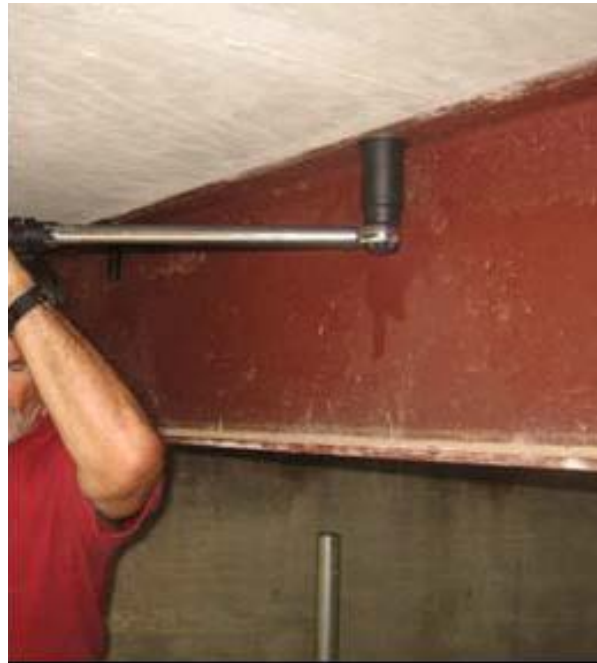
Fig. 5.12: Tightening of nut to specified torque
